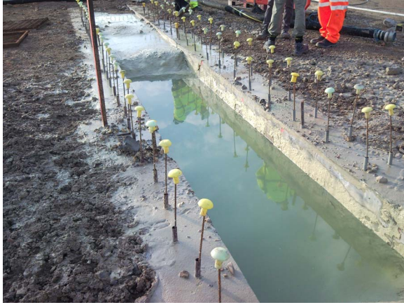
Figure 1 Bleed water in trial panel
