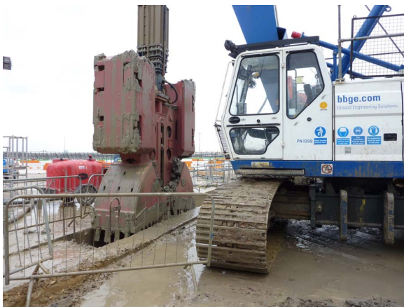
Figure 3 Diaphragm wall rig
