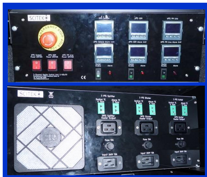
Figure 20 Photographs of back panel and front panel of 3 channel heater control unit
