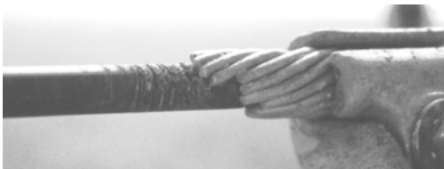
Fig. 3. Damage on a polyethylene sheathed cable in Chile on a 100 kV line. The metallic wires are part of the clamping system and the galvanised clamp around those wires attaches the vibration damper.
