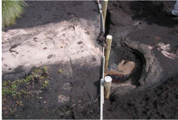
Figure 2.12 Water erosion in front of a wooden dam. Sediment is still held behind dam, as scouring has not yet reached bottom of dam.
