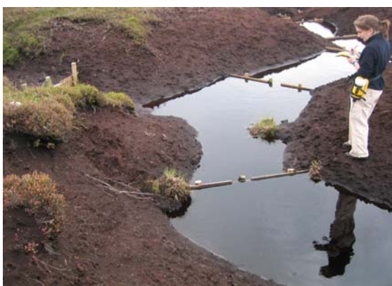
Figure 2.10 (left) Wooden piling on Kinder Scout is strong enough to hold water as well as plastic piling
