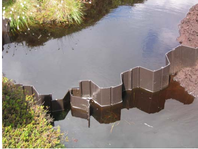
Figure 2.4 Plastic dam on Within Clough. Gully sides range from well established dwarf shrub, Eriophorum patches and bare peat.
