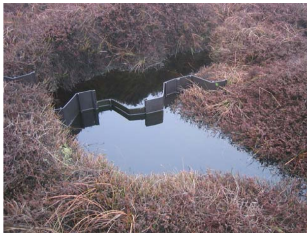
Figure 2.8 Plastic dam on North Grain. Gully sides are generally well vegetated with established dwarf shrub and Eriophorum patches, but locally bare peat is present. The banks provide a good source for plant colonisation by e.g. rhizomes.
