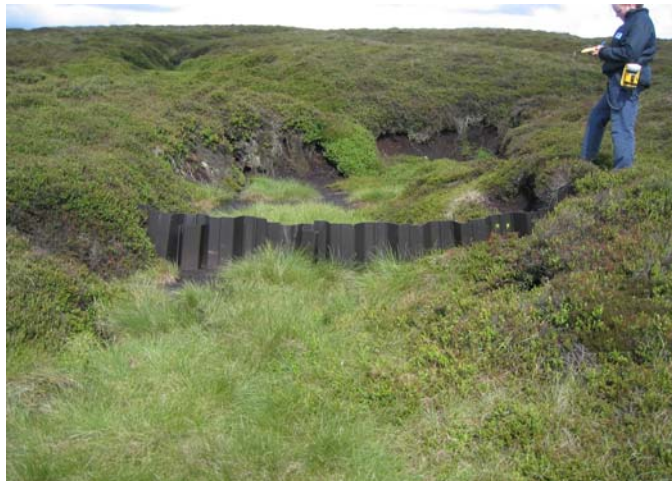
Figure 2.5 Eriophorum angustifolium behind plastic dam at top of gully. This dam was installed in a vegetated area possibly to protect the already established vegetation or to prevent upstream erosion.
