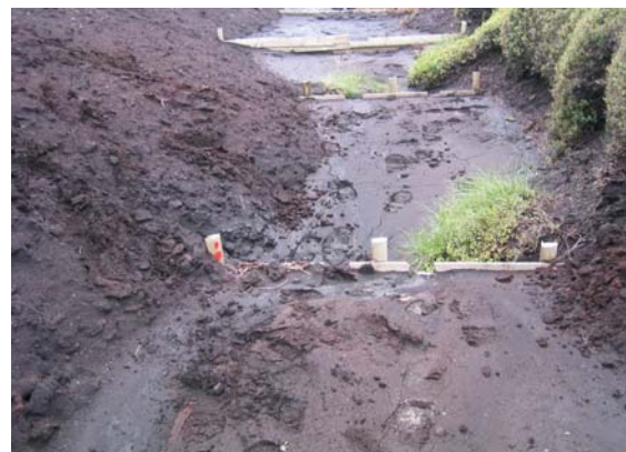
Figure 2.10 (left) Wooden piling on Kinder Scout is strong enough to hold water as well as plastic piling
