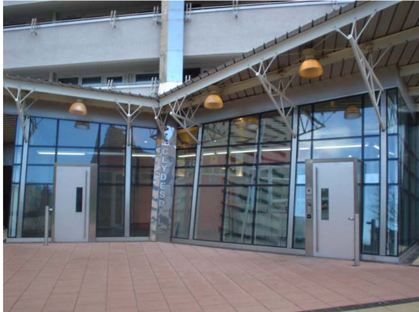
Photo 2.5. The refurbished entrance of Clydesdale, one of the Sentinel Towers; after refurbishment the area around the towers has been fenced and a doorman was introduced to improve safety and services.
