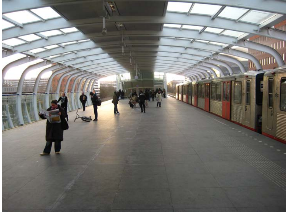
Photo 5.4 Refurbished elevated train station
