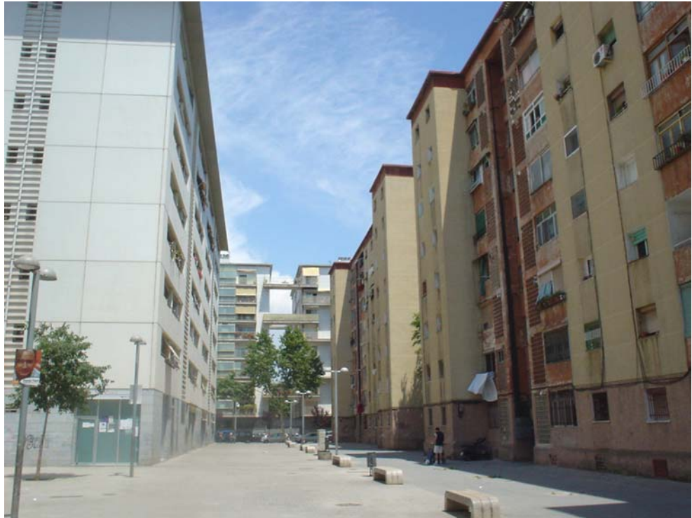
Photo 4.4. Regeneration in Sant Roc. Left, the newly developed apartment buildings and, right, the apartment blocks to be demolished
