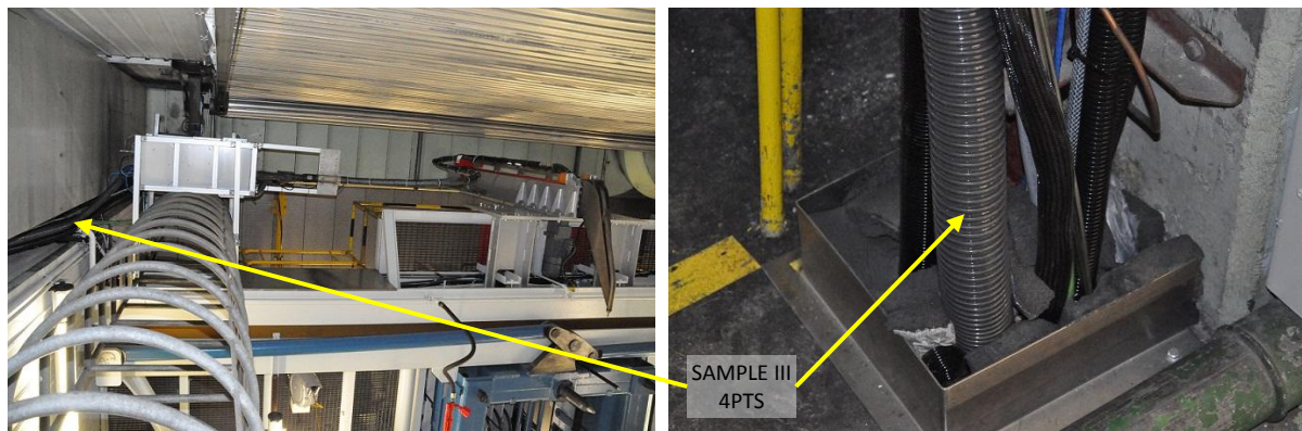
Figure 45 Installation of SAMPLE III 25m PTFE sample line (4PTS)
