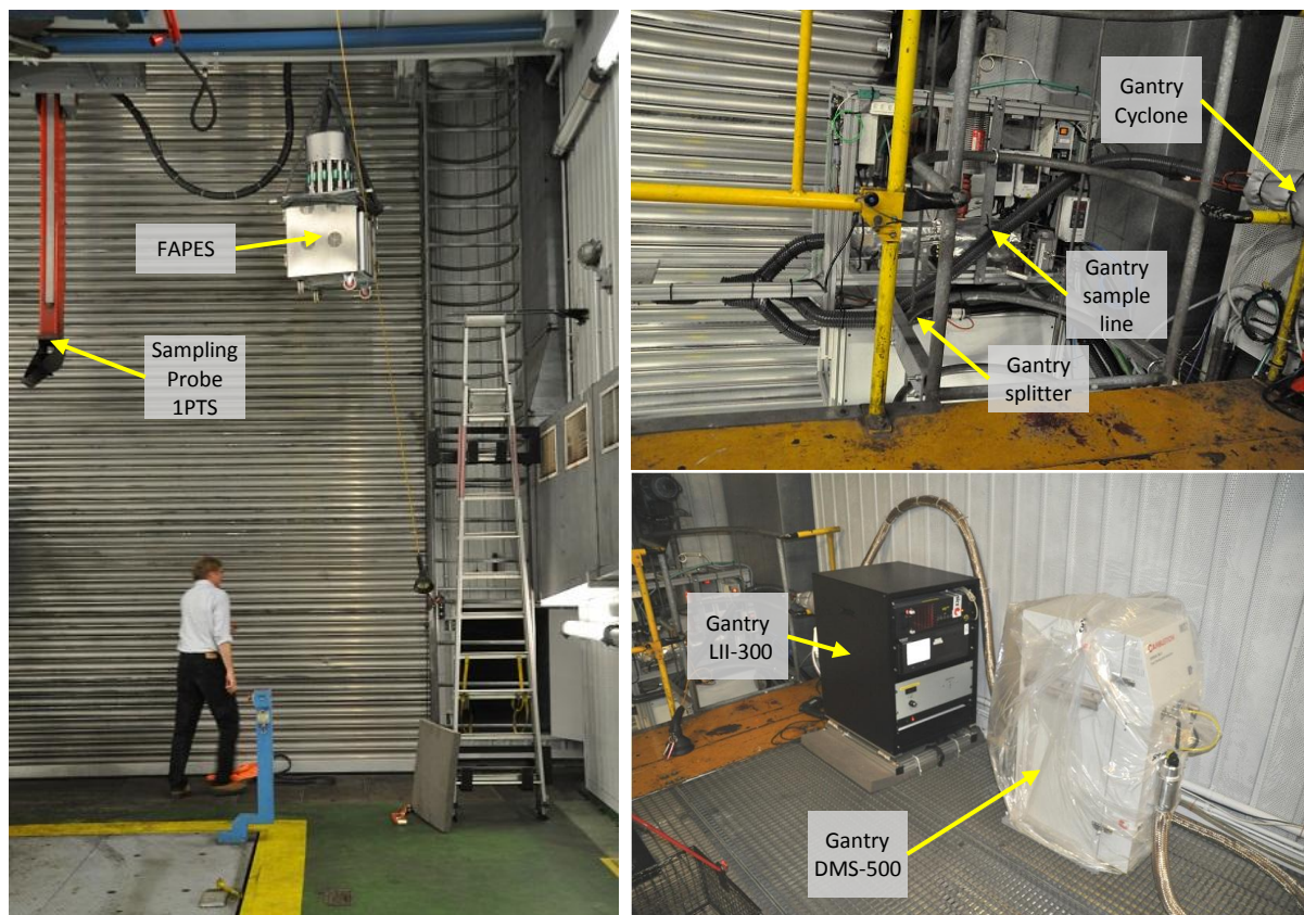
Figure 49 Installation of the Gantry instruments
