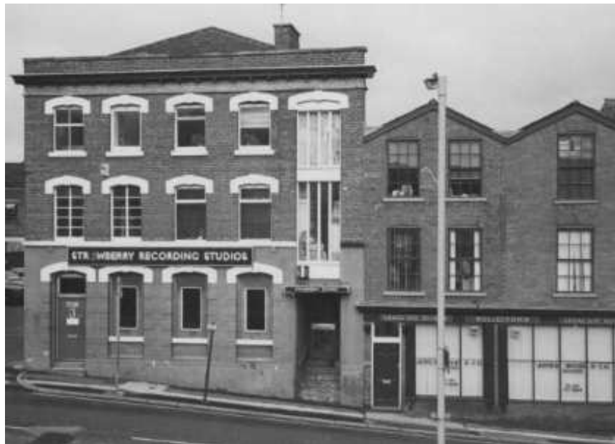
Figure 53: The Strawberry exterior in the 1980s, particularly showing the steep slope 28
