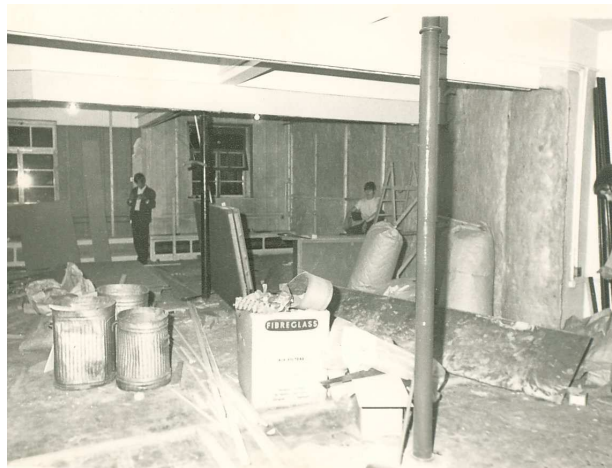
Figure 3: Work begins at Waterloo Road (with Eric Stewart far right) 158
