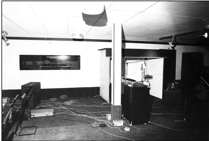
Figure 30: Wires and cables in Strawberry's recording area in the early 1970s 79
