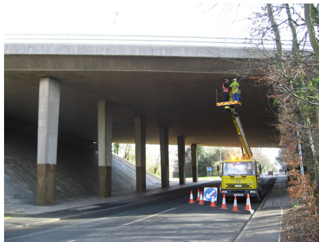
Figure 4. Ferriby Road Bridge (Photograph: Dr P. J. Bennett)
