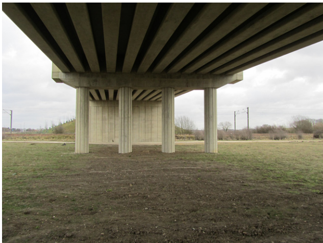
Figure 2. Nine Wells Bridge, Cambridgeshire (Photograph: Authors)
