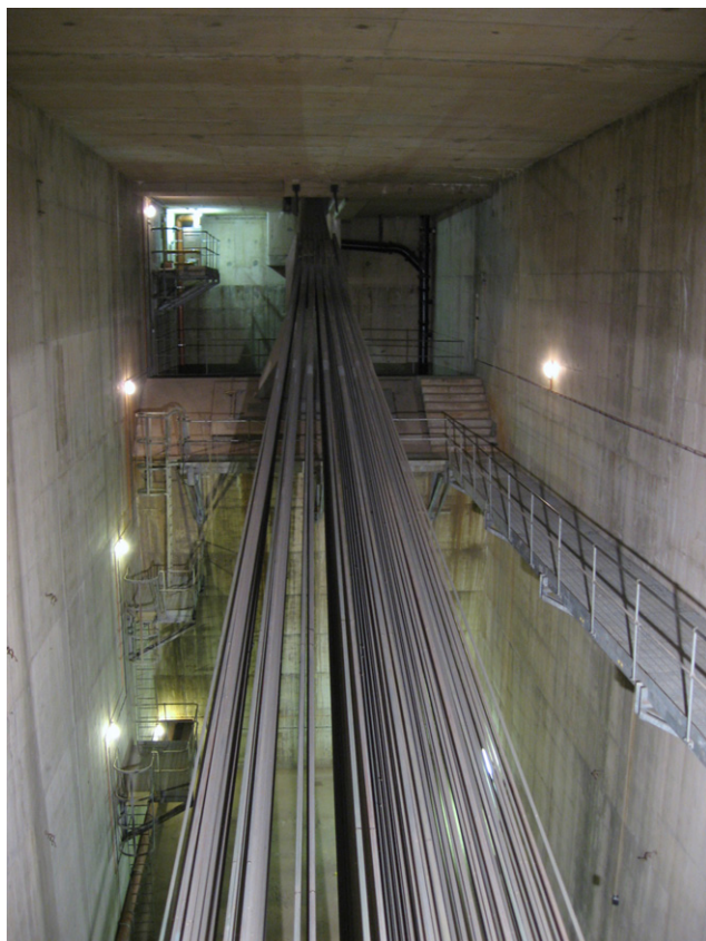
Figure 3. Humber Bridge: Hesse Anchorage (Photograph: Dr P. J. Bennett)
