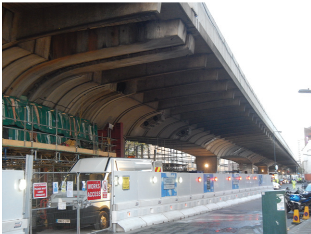
Figure 5. Hammersmith flyover (Photograph: Authors)
