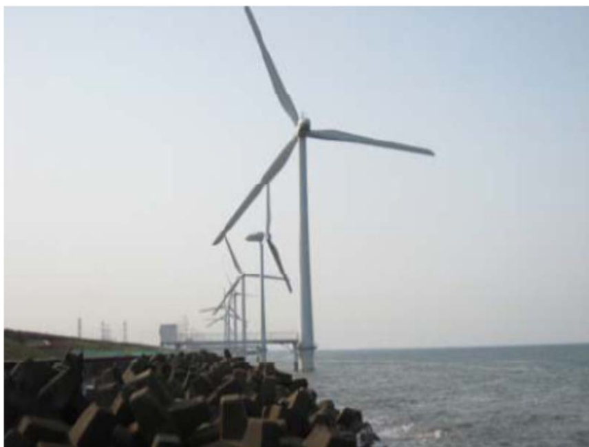
Figure 2: Photograph of the Kamisu (Hasaki) wind farm following the 2011 Tohoku earthquake
