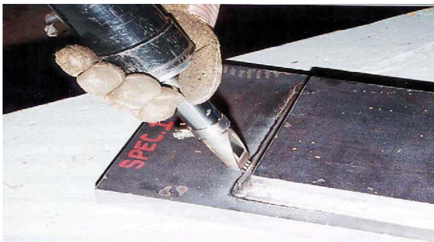
Figure 8: Ultrasonic peening being applied to a steel weld toe [91].
