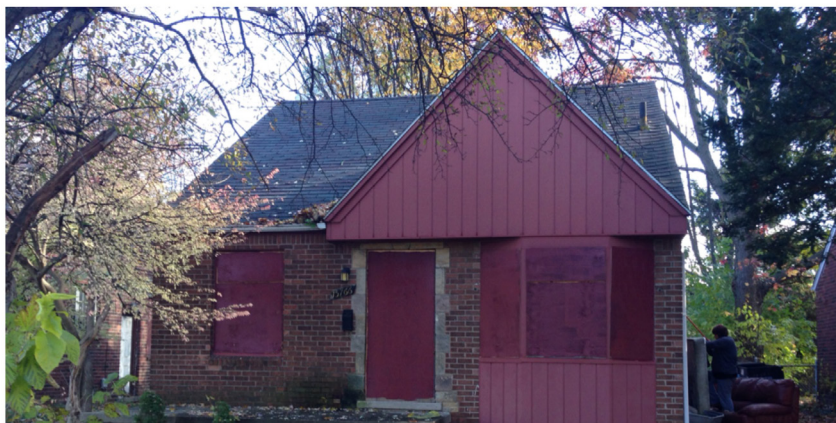
Fig.9.1 and 9.2: Before and After Repair
