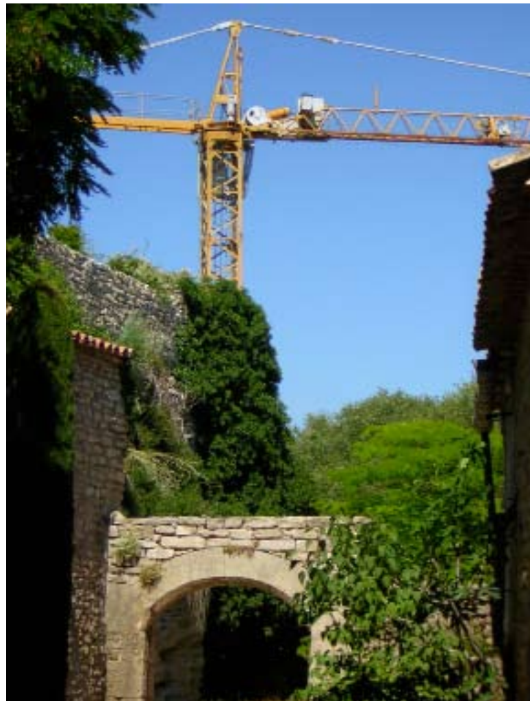
Construction crane in Goult, France. Photo: Sarah Elizabeth Ross
