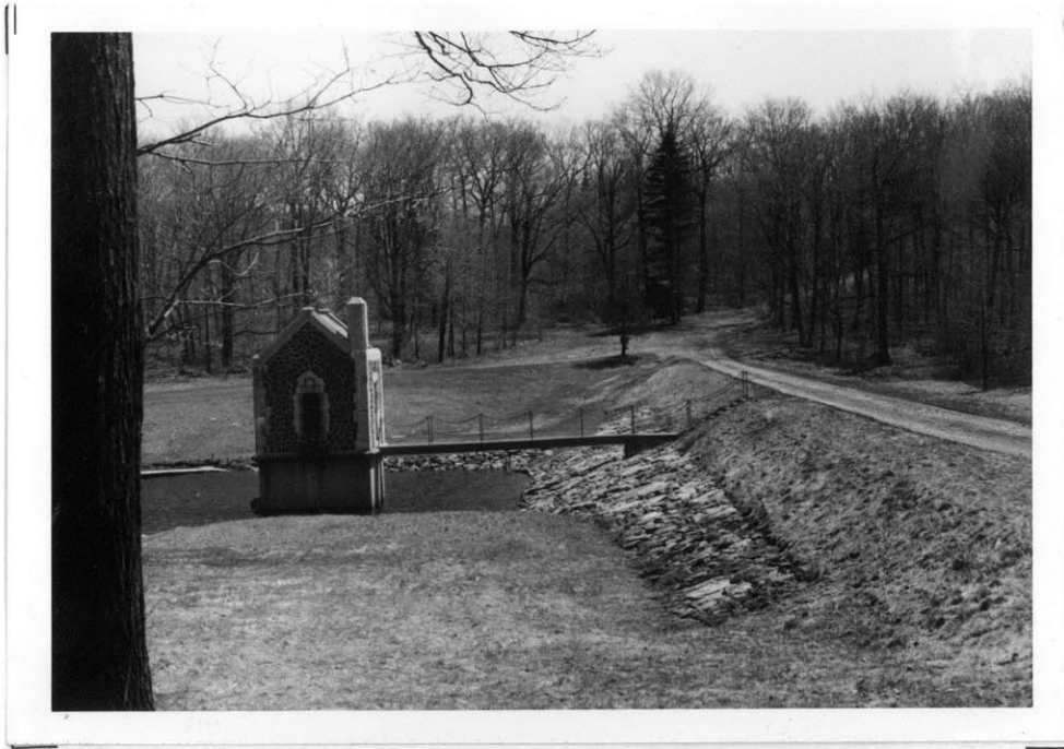
Figure 4.5 Bank of Echo Lake at the Pump House
