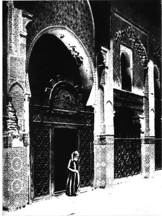
PARTIAL COMPLETION; PLACE DEFINITION IN LARGER DIRECTIONAL ORDER... MOROCCO
