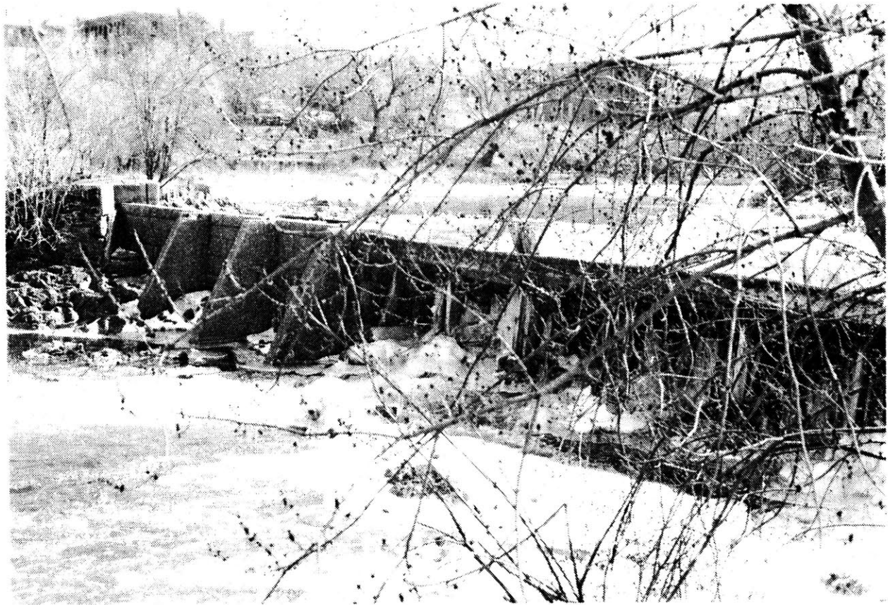
Middlesex Co. Dam
