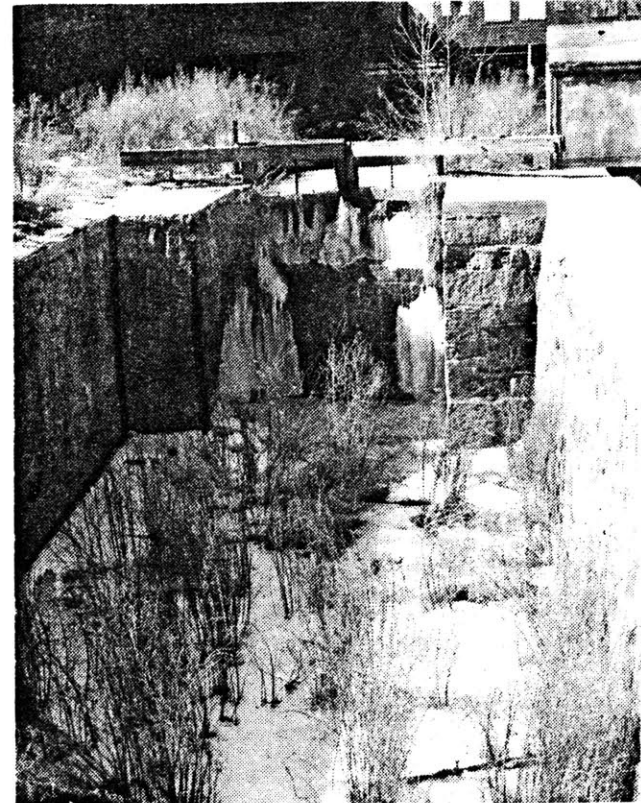
Boat lock adjacent to site
