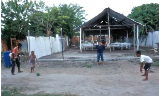
Baru: IPUC before the restructuring works
