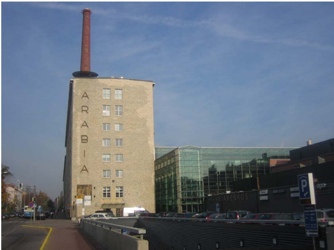
Figure 1: Former Arabia porcelain factory (now University of Art and Design Helsinki)
