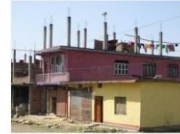
Newly constructed concrete house
