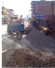
Construction workers dropping off gravel
