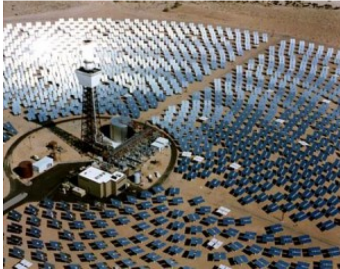
Figure 2.4: The anticipated completed solar project located in the Mojave Desert [8]
