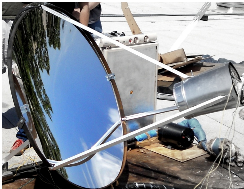
Figure 3.8 – Final Construction of New Solar Tracker
