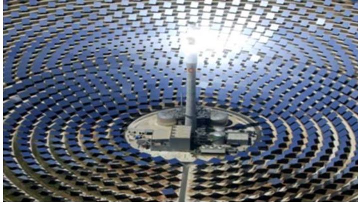
Figure 2.1: Industrial Scale Concentrated Solar Plant
