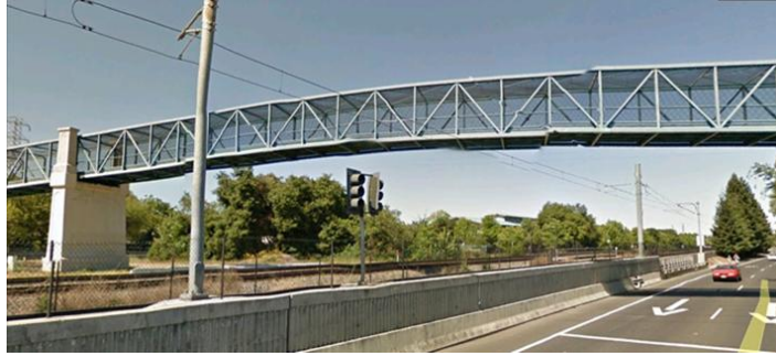
Figure 2: Mountain View Caltrain pedestrian bridge
