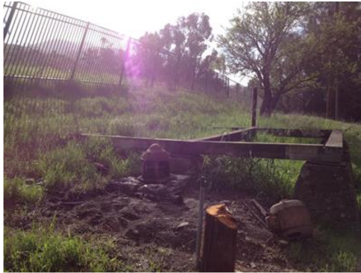
Figure 18 –Photo after demolition of shed encompassing turbine pump
