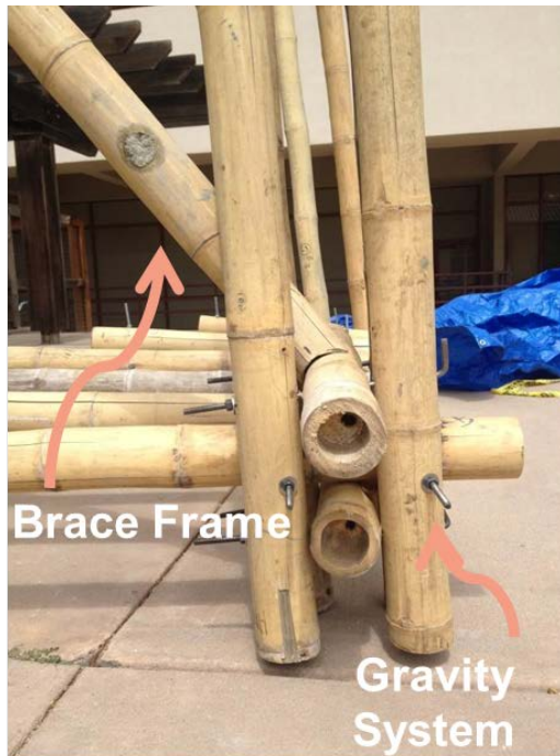
Figure 23. Fully constructed brace frame integration
