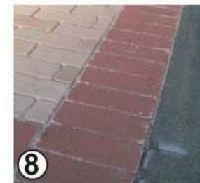
⑧ "B" and "C" Terrace Paving: Pattern Paving Products colored and stamped asphaltic concrete paving, or equal (see colors below)
