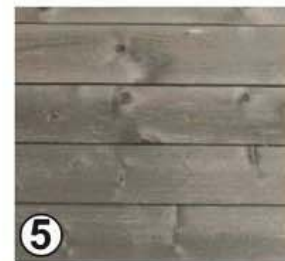
⑤ Patio Fences: 1 x 8 cedar or redwood boards, unfinished (will weather to silvery-grey)
