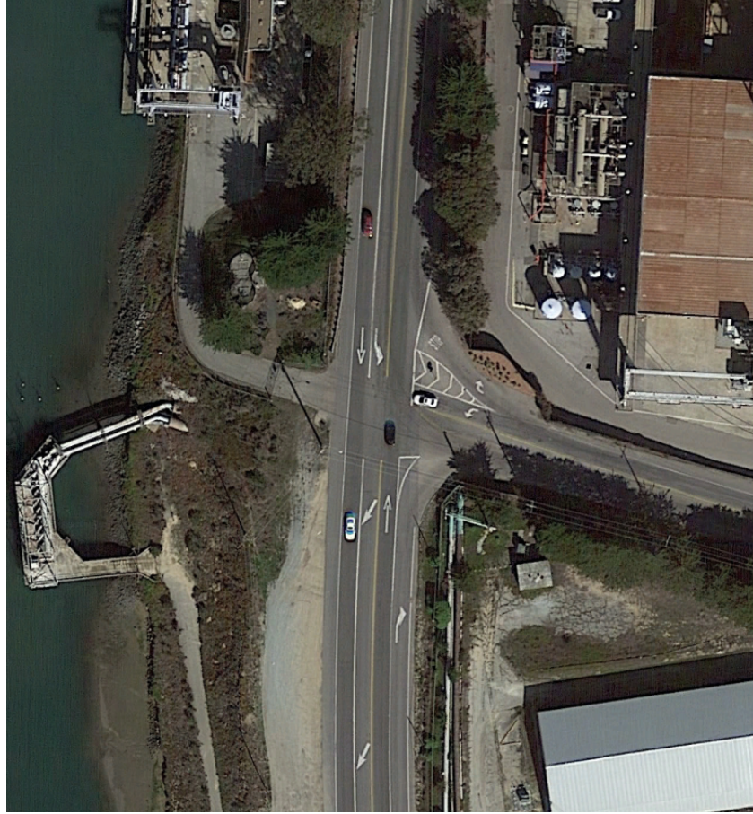
Figure 3: Existing conditions at Highway 1 at Dolan Road in Moss Landing. (North up)
