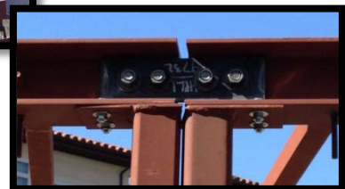
FIG. 7 - 2013 RADIANT HOUSE MODULE CONNECTION
