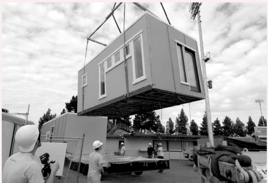
Team members look on as the Solar Decathlon house is loaded on the trailer.
