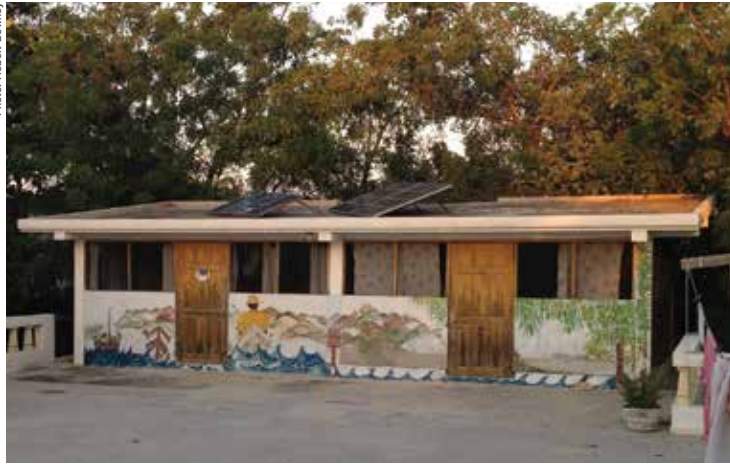
Newly installed solar panels serve the medical/dental clinic well.
