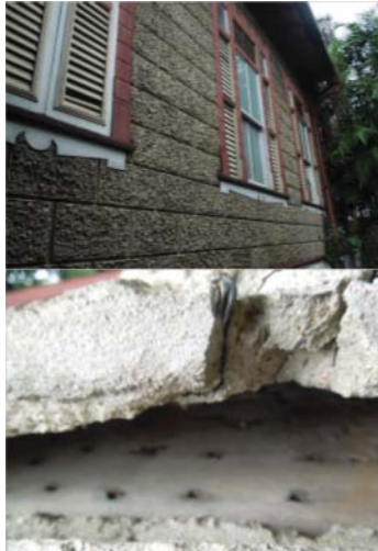
Figure 10. Side façade of the Boissière House. In this photo some of the plasterwork is removed to show the use of nogging below. By L. Welcome, Jan 2010.
