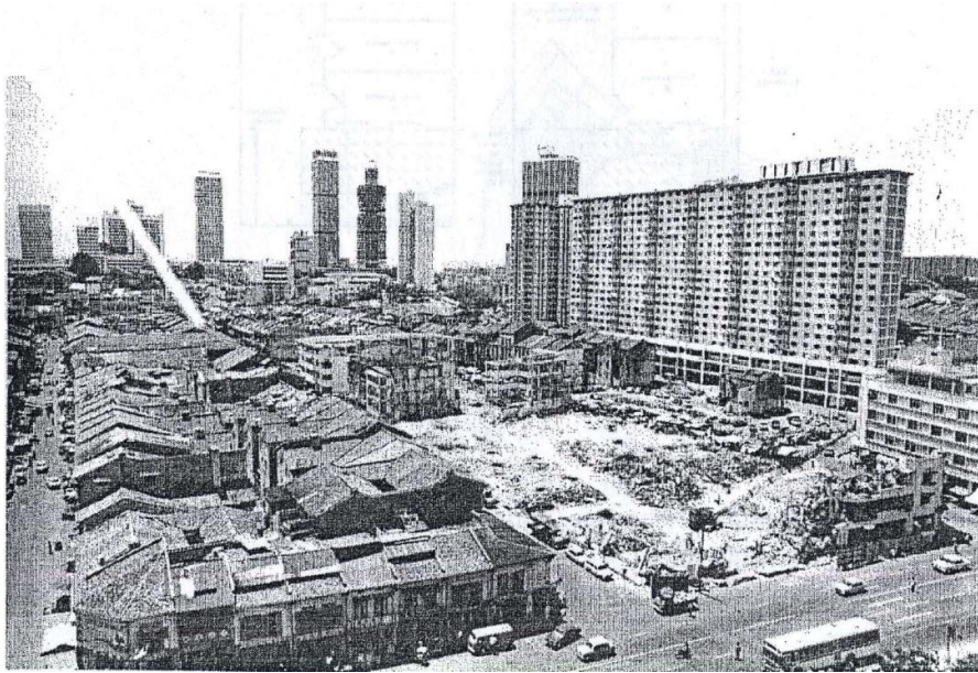
FIGURE 19. Replacing shophouses with tower blocks in Singapore "Evolution of the Chinese Shophouse on the Malay Peninsula," 70.
