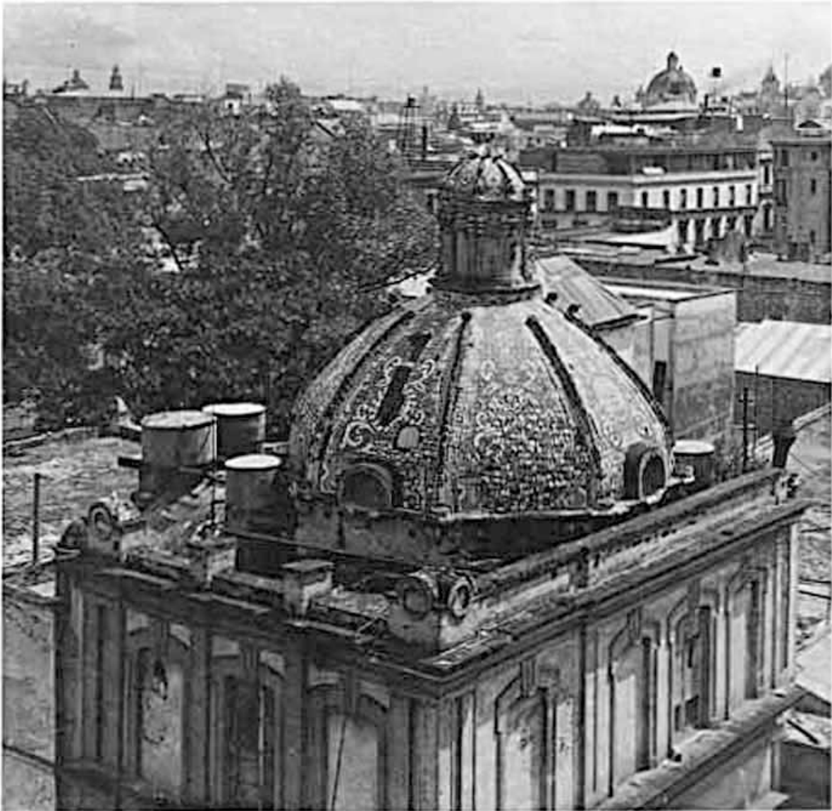
Figure 34: The San Antonio chapel still exists as a bookstore, isolated from the remaining fragments of the convent.
