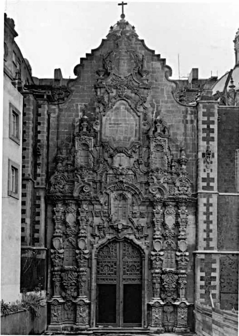
Figure 27: Façade of the Balvanera Chapel as it stands today, after its defacement by the Protestant minister. Source: Tovar de Teresa, City of Lost Palaces , 25.
