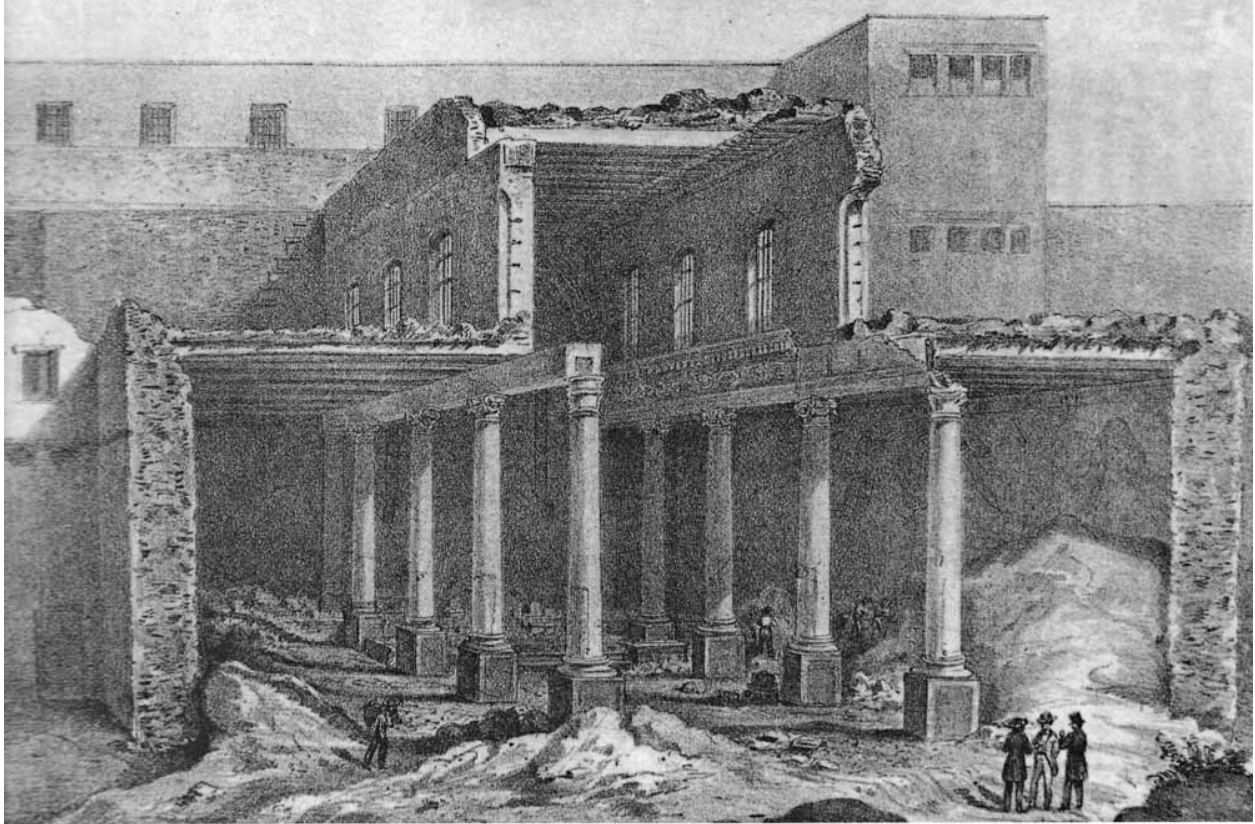
Figure 20: The Chapel of the Servites that had once been the Chapel of San José de los Naturales; the great open chapel was reduced from its original seven naves to five, and eventually to only three. Its open façade was closed at this time and renamed. Source: Tovar de Teresa, City of Palaces , 19.
