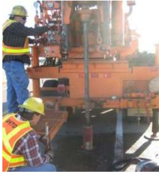
Figure 3.19. Coring by Arkansas State Highway and Transportation Department (AHTD) personnel for installation of two stage borehole test casing.
