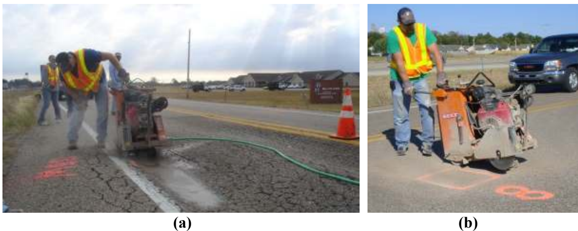
Figure 3.3. Two foot by two foot test sections cut by Arkansas State Highway and Transportation Department (AHTD) personnel using a wet concrete saw a) Section 13W and b) Section 8.
