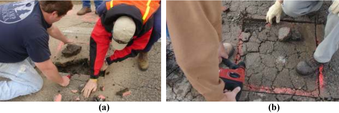
Figure 3.5. Removal of asphalt using a) crowbar (Section 13W) and b) hammer drill (Section 13BW).
