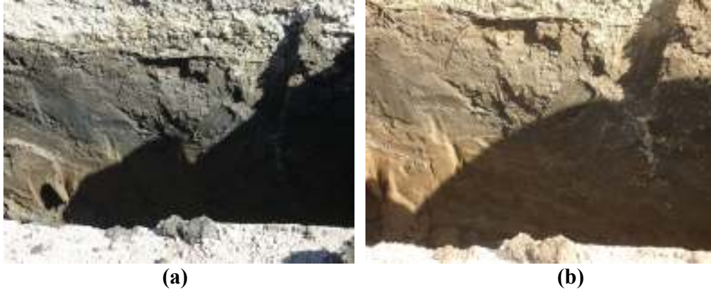
Figure 4.33. Discoloration in subgrade soil in Section 13BW after trench excavation on the a) east side and b) west side of the trench.
