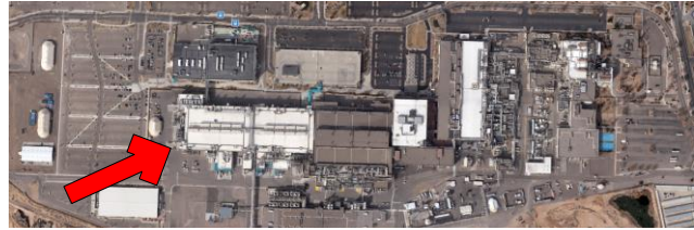
Figure 10: Intel utilities building.
