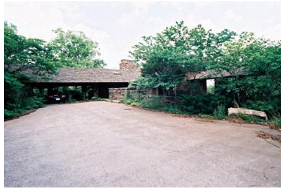
Figure 50: Walton House, driveway
