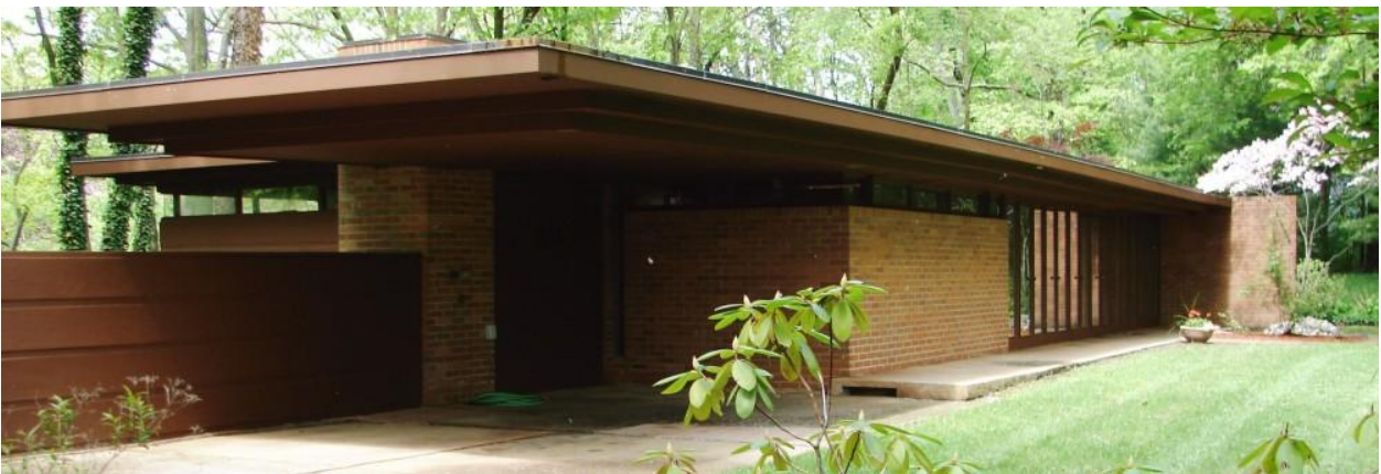
Figure 28: Goetsch-Winckler House, Exterior Photograph showing the carport and overhanging roof.
