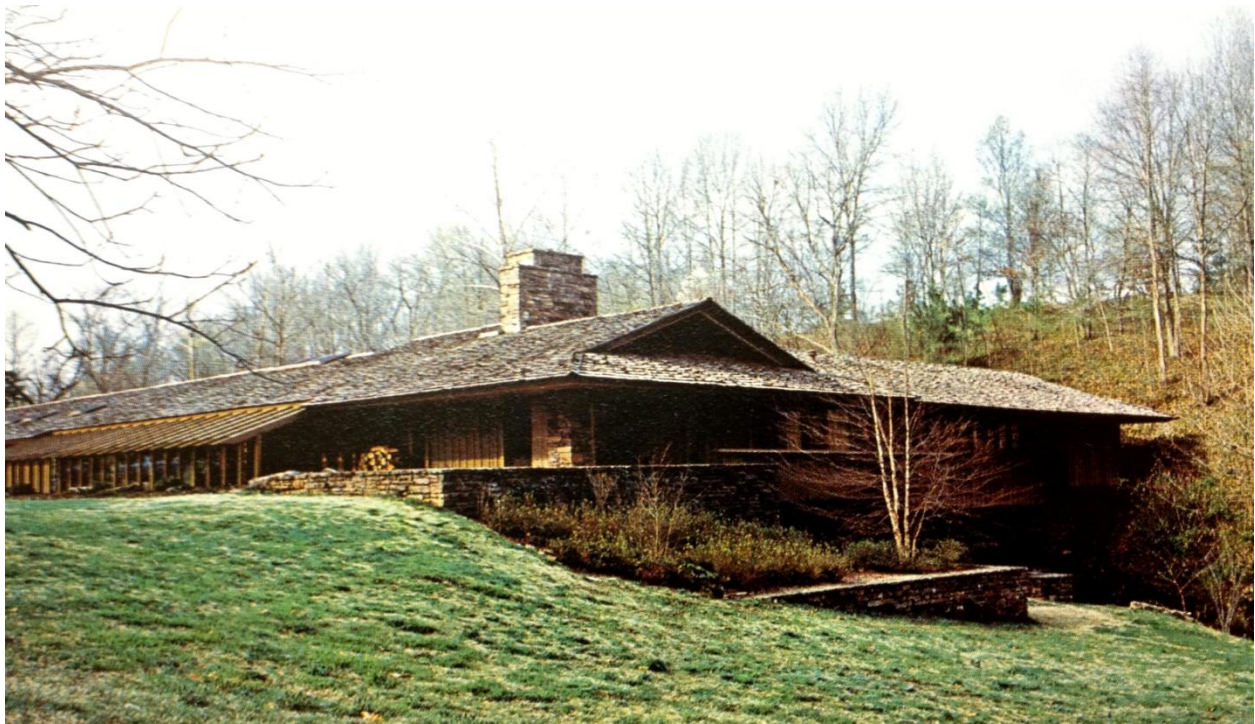
Figure 47: Walton Residence, Exterior
