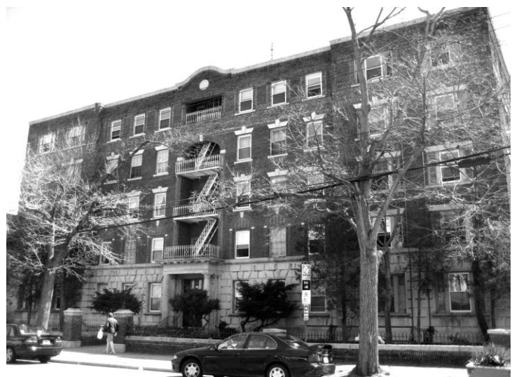
Figure 5. STONE FAÇADE, THE KNICKERBOCKER (625-635 ORANGE) Source: Photograph taken Spring 2007 by author
