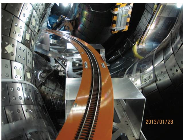
FIG. 6. Test installation of track inside the LHD vacuum vessel that will be used for in situ NFM calibration.
