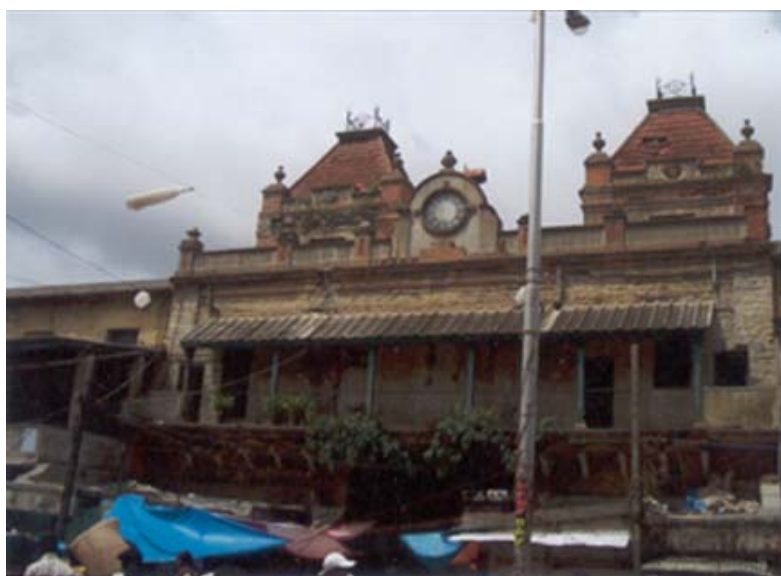
Figure 2. Old hatched asbestos building at K. R. Market.
