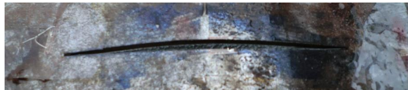
b) Fracture area in SP1-D4-L100
