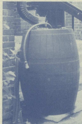
Rain barrels are an easy way the community can reduce urban stormwater runoff.
