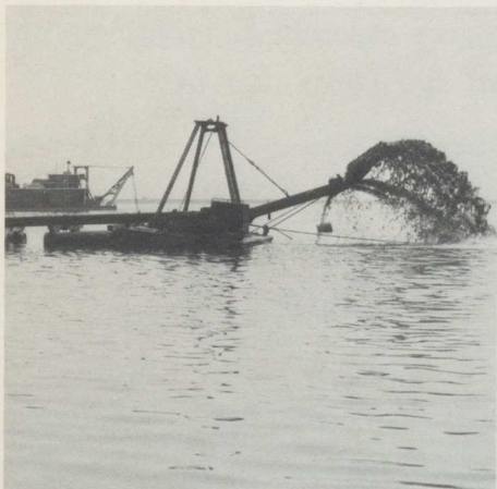
Dredging in the St. Clair River.
