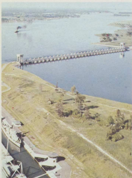
Iroquois control works.
