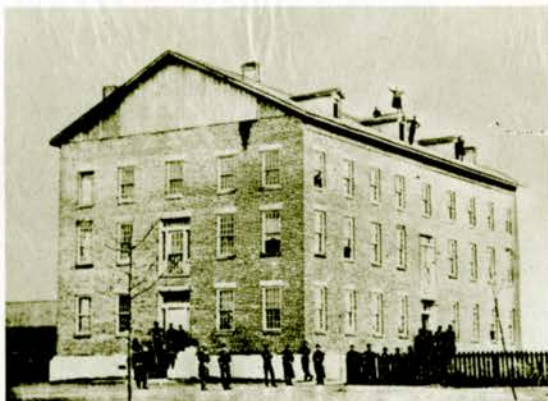
The original Assumption College, built in 1857 and demolished in 1965, garrisoned British troops during the Fenian Raids.
