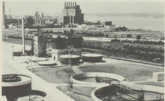
A waste treatment plant for a modern industry safeguarding water quality.
