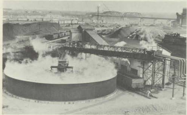
Treatment of chemical wastes to prevent tastes and odours in water.
