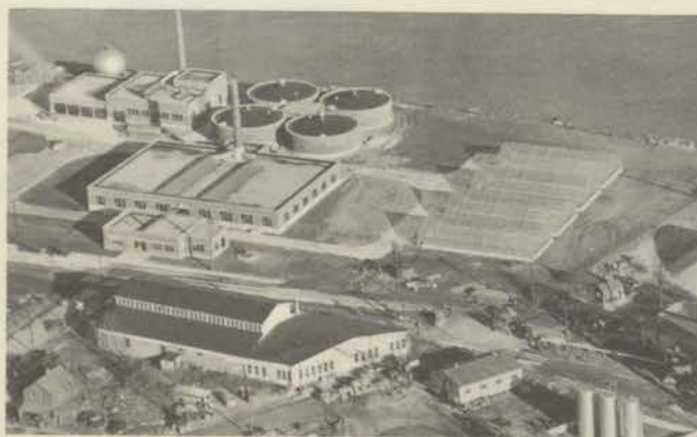
Many sewage treatment plants have been built in this period.
