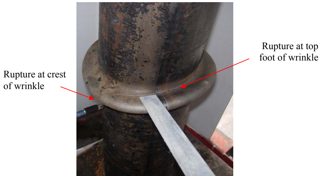
Figure 4.14: Two large cracks appeared after pressure test
