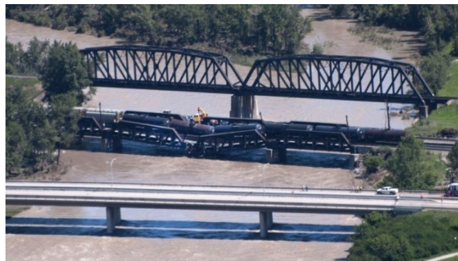
Figure 1.2. Derailed train in scour-related bridge collapse in Alberta (CTV News, 2013)
