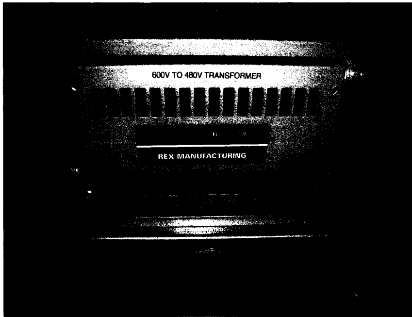
Figure 52: Rex Manufacturing Auto-transformer.
