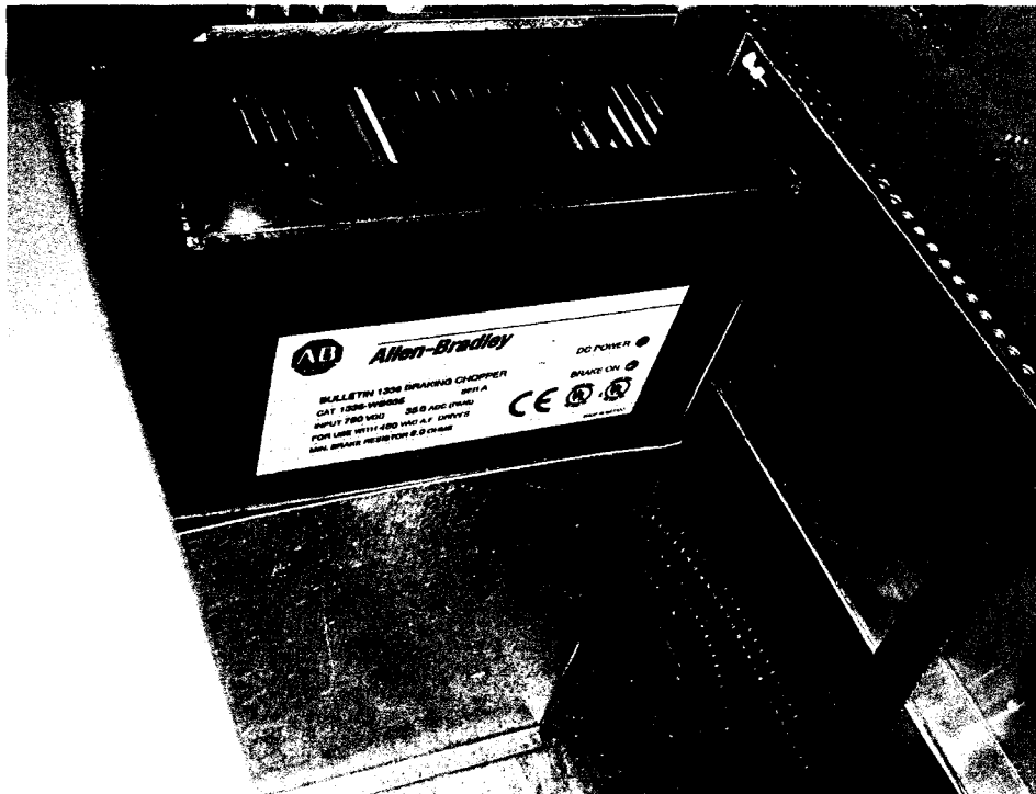
Figure 51: Allen-Bradley Dynamic Braking/Chopper Module.
