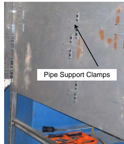
d. Liquid handling system panel construction-2
