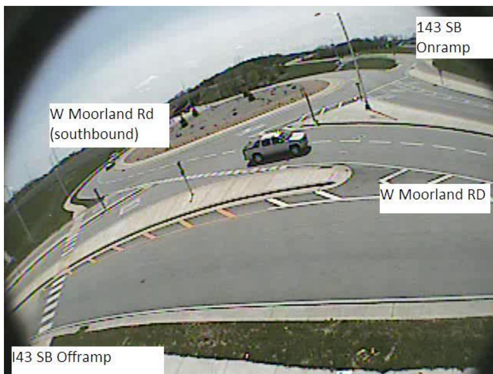
Figure B-8. Moorland North Roundabout Screenshot
