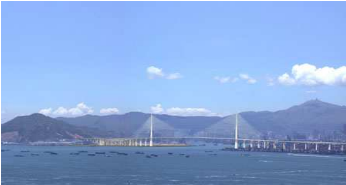
Figure 4-6 View of Stonecutters bridge at the entrance to the Kwai Chung container port
