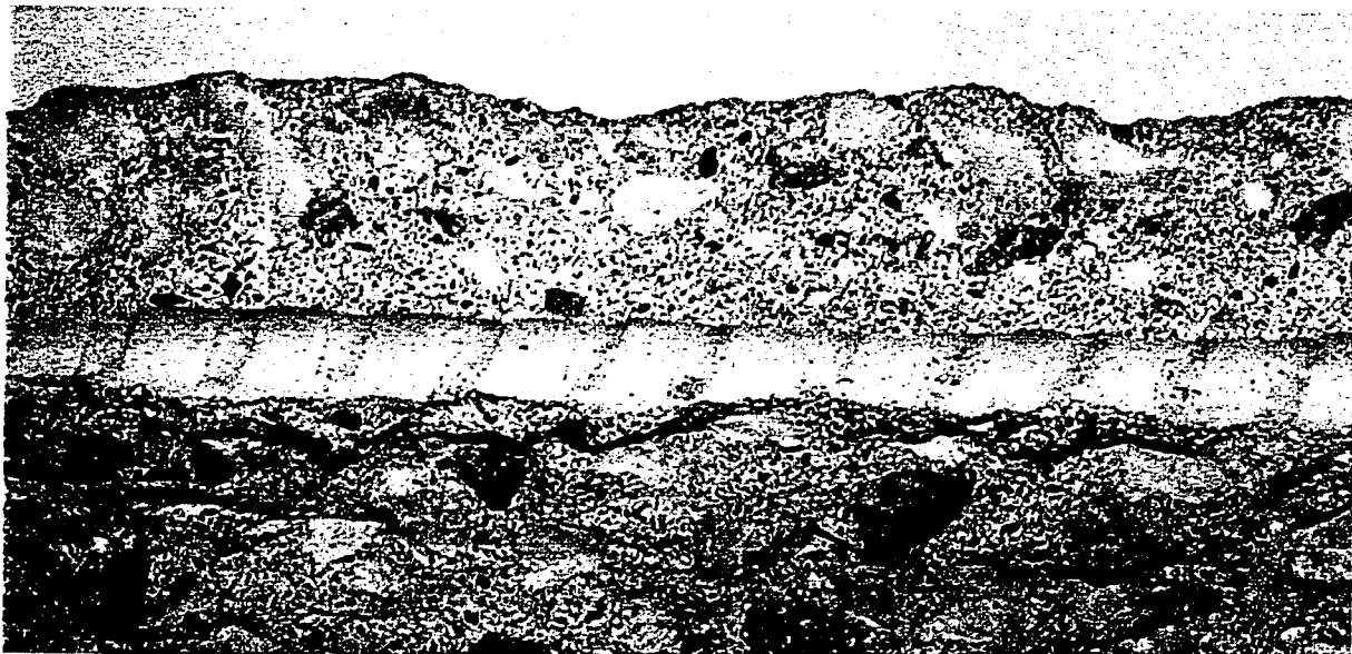
Figure 5.2: Appearance of concrete cover of beam reinforced with D1-D9.70 CFRP bar
