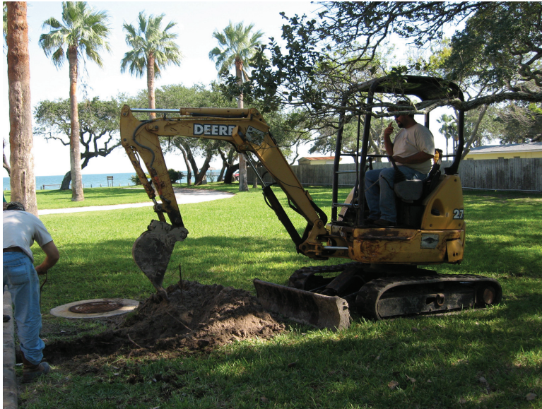
Figure 4-12. Mechanical trench excavation.
