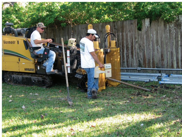
Figure 4-9. Horizontal line boring.
